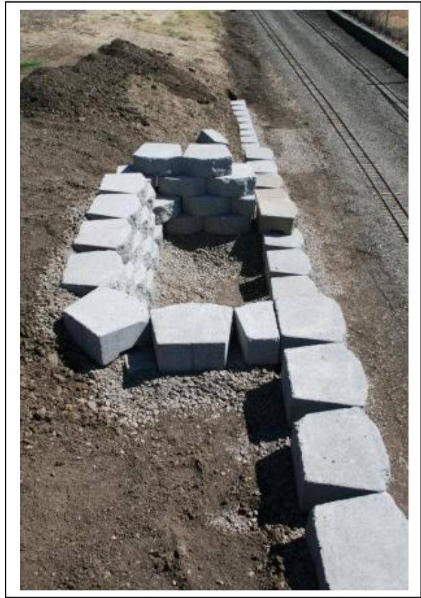
These images were taken on July 23 rd . At that time Elvin was into his fourth day of positioning the blocks for the new retaining wall. This design of this wall will also feature “planter box” areas for low maintenance shrubs and flowers. This is a great improvement to our layout.
