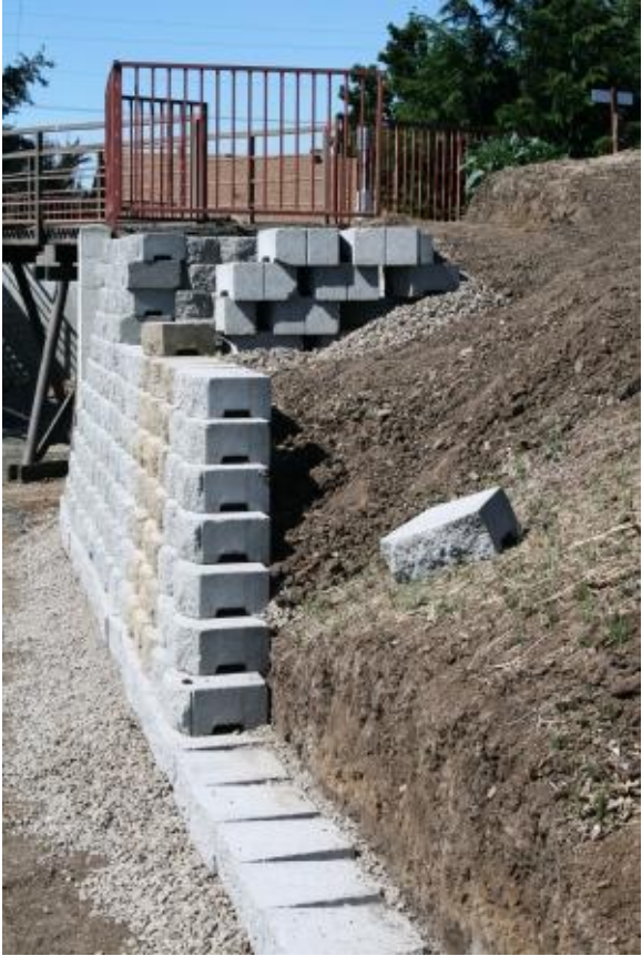
These images were taken on July 23 rd . At that time Elvin was into his fourth day of positioning the blocks for the new retaining wall. This design of this wall will also feature “planter box” areas for low maintenance shrubs and flowers. This is a great improvement to our layout.
